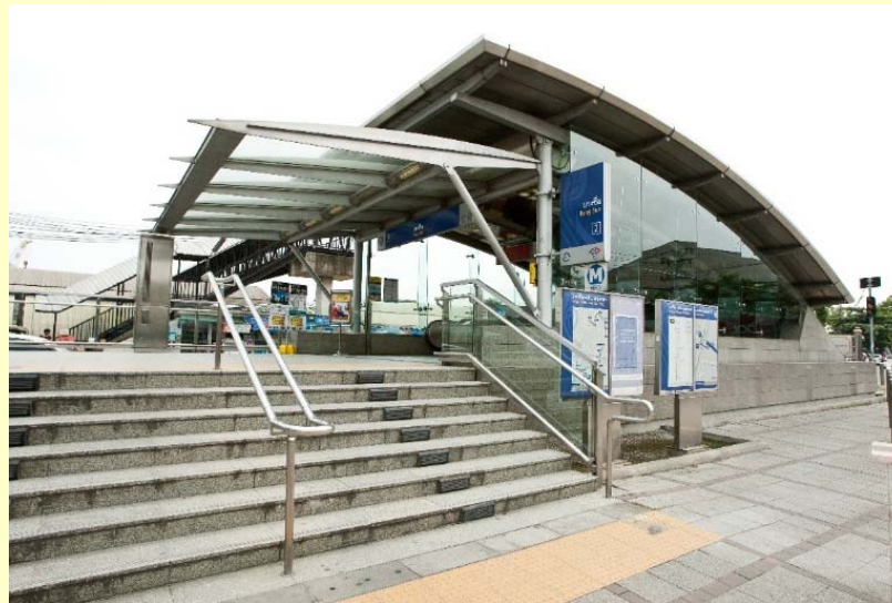
Subway that is resistant to flood (Photo: Shinichi Kubo/JICA)
