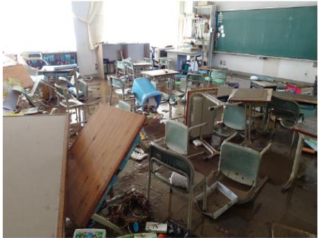
School facilities damaged by the inflow of earth and sand due to heavy rain.
