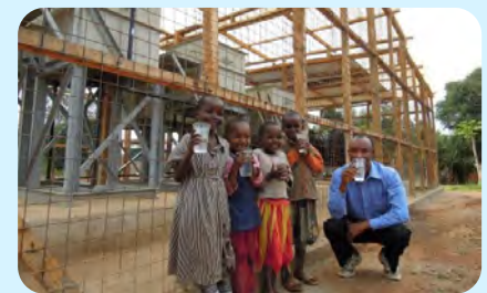
Local residents hold clean water in front of a "Slow Sand Filtration system"
